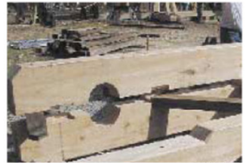
Joel McCarty Main beam before assembly around mast. The circular aperture closes around a necked-down portion of the mast to form a pivoting joint, hardened by steel bearing surfaces not yet applied. See also photos on page 16.
