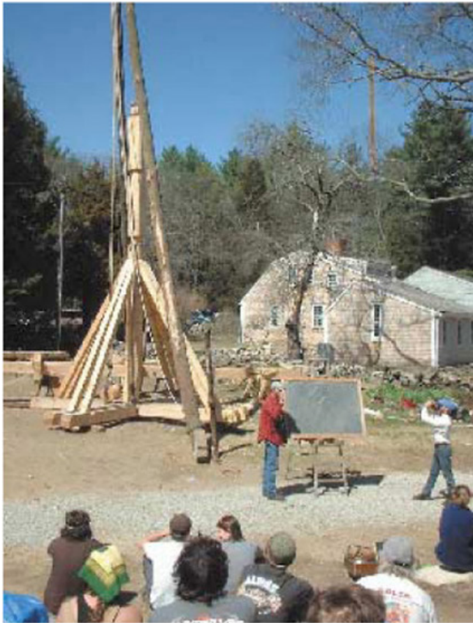
Virginian and fly fisherman Al Anderson, henceforth to be known as Professor Lift, explains to the crew what's going to happen now that the base and mast have been made ready to receive the rotating assembly.
